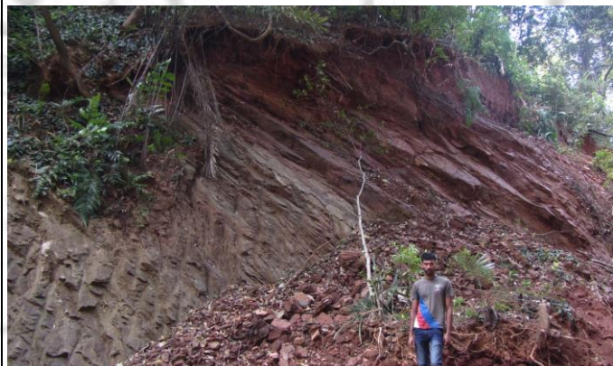
Photo-6: Planar wedge failure in schist near Sasiguli, KAR/UK/48J11/2014/16.
